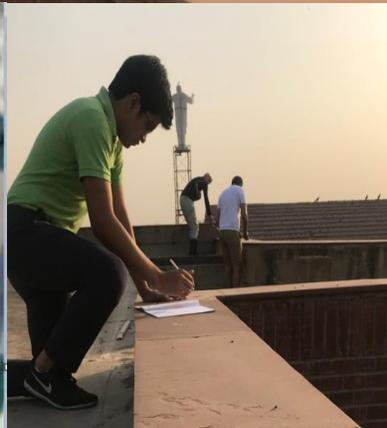
Measuring the available roof top area at Deepashram, noting the direction of the sun and planning for the layout of the panels required for 19.5 kW.
