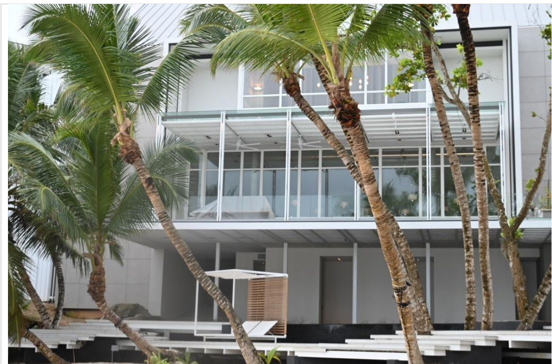
Figure 14. New main public area which is different from the original master plan. Large picture window need to be fitted with automatic opaque blinds, curtains, and tinted glass.
