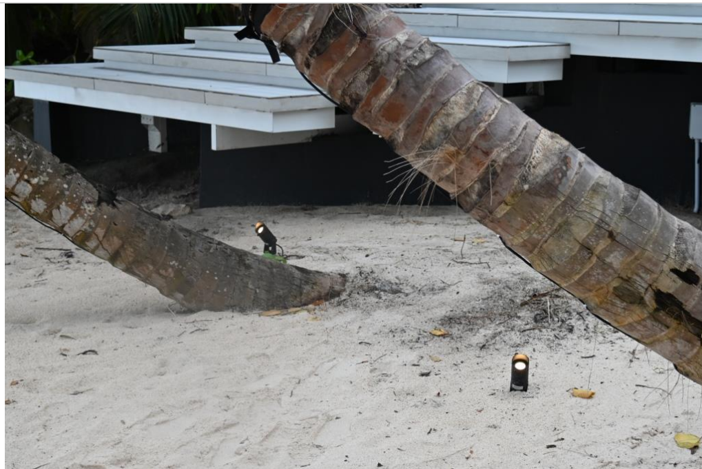
Figure 16. Upward directed luminaires such as those shown in this photo are inappropriate in the vicinity of a turtle nesting beach. They need to be removed.
