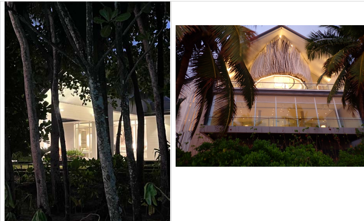
Figure 19. Virtually all of the buildings on the property are light-coloured and reflective , producing Skyglow . Ideally the outer walls of the buildings should be darkened or in some way made less reflective (for example by using stucco, or a matte finish).
