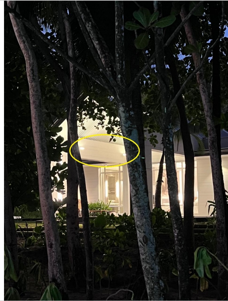
Figure 17. The luminaires indicated in this photo are primarily decorative and serve no practical purpose.
