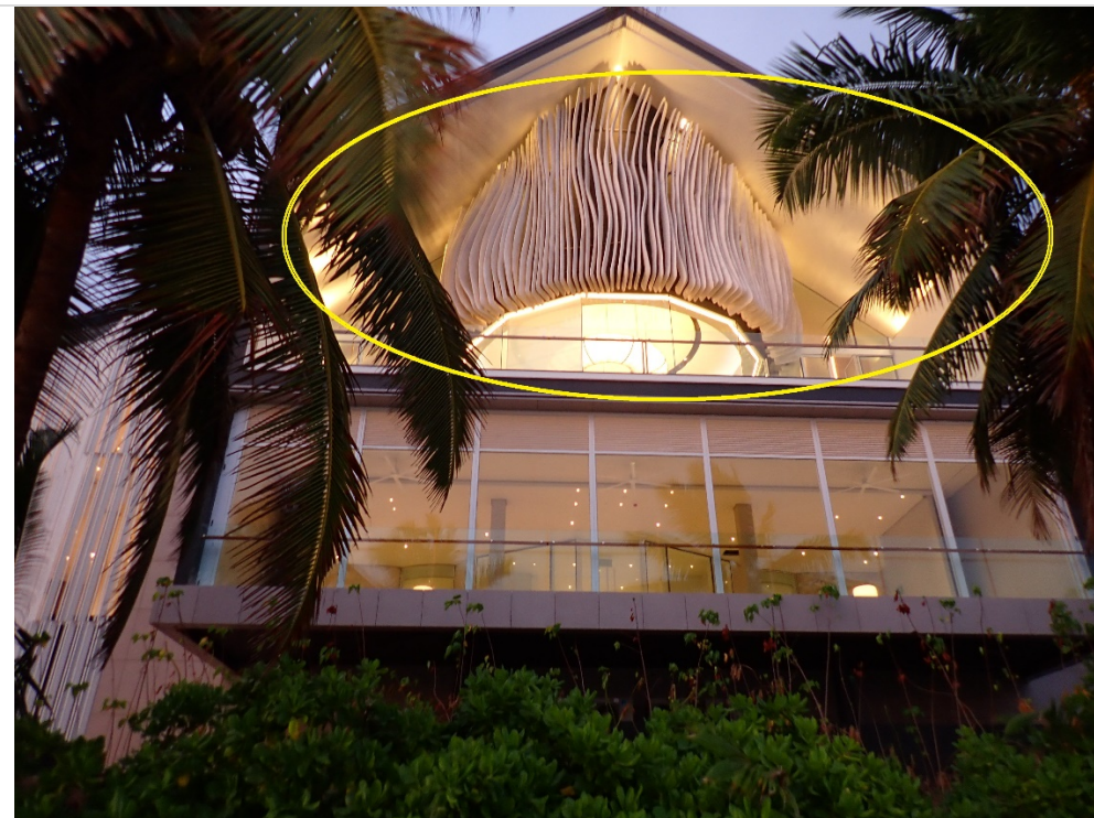
Figure 18. All the lights associated with the second floor of this building need to be turned off after sunset until before sunrise. They are purely decorative and disruptive.
