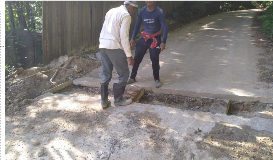
22b. Road "bridge"
