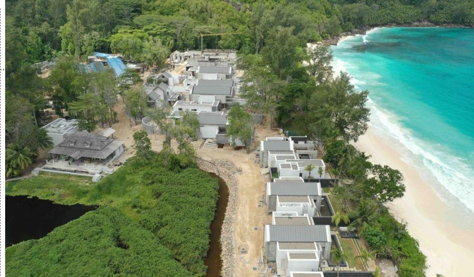
50b. New access to beach villas wider and closer to the wetland
