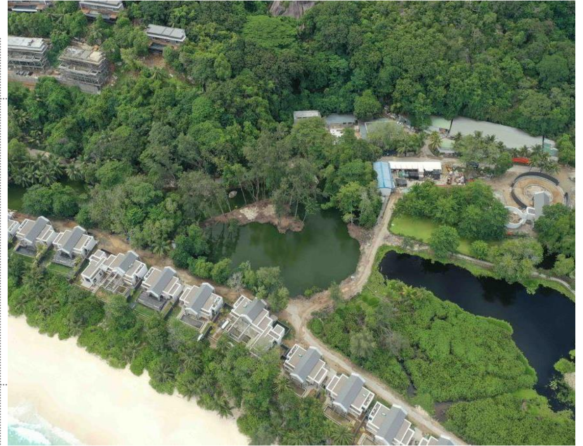
2b. New main access road through the wetland
