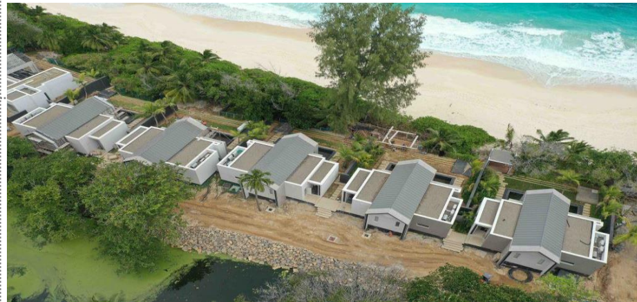
50c The wetland banks no longer natural but artificial rock embankments
