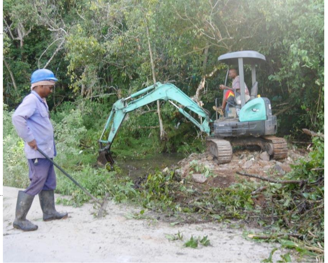
57b Desilting by excavator
