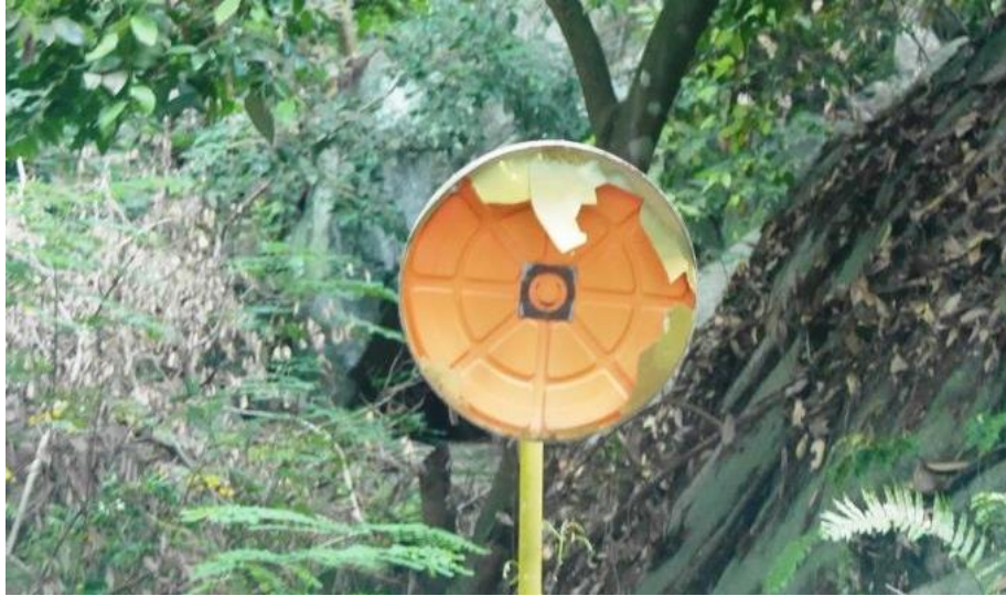
35a Lack of functional blind corner mirrors
