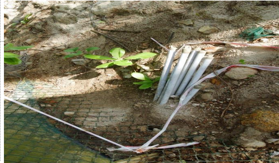
43c This looks like power conduits going out to the beach. Is there beach lighting planned?
