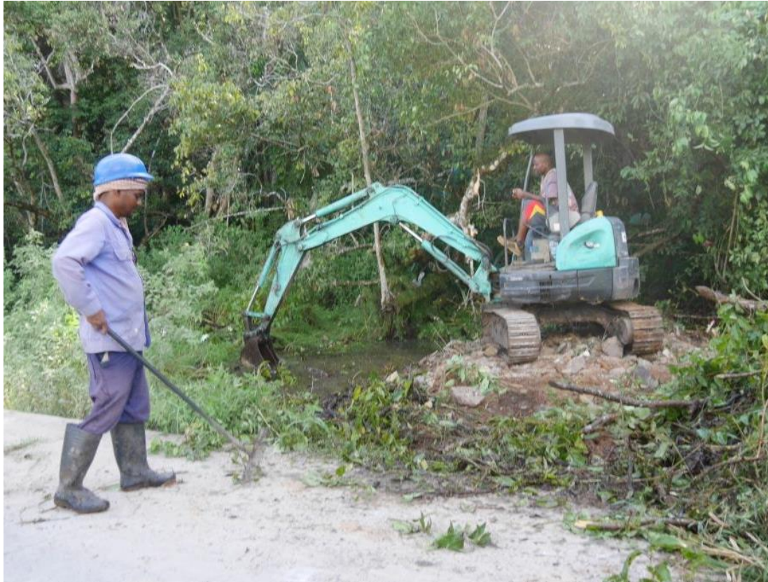
9a. Heavy machinery in the wetlands
