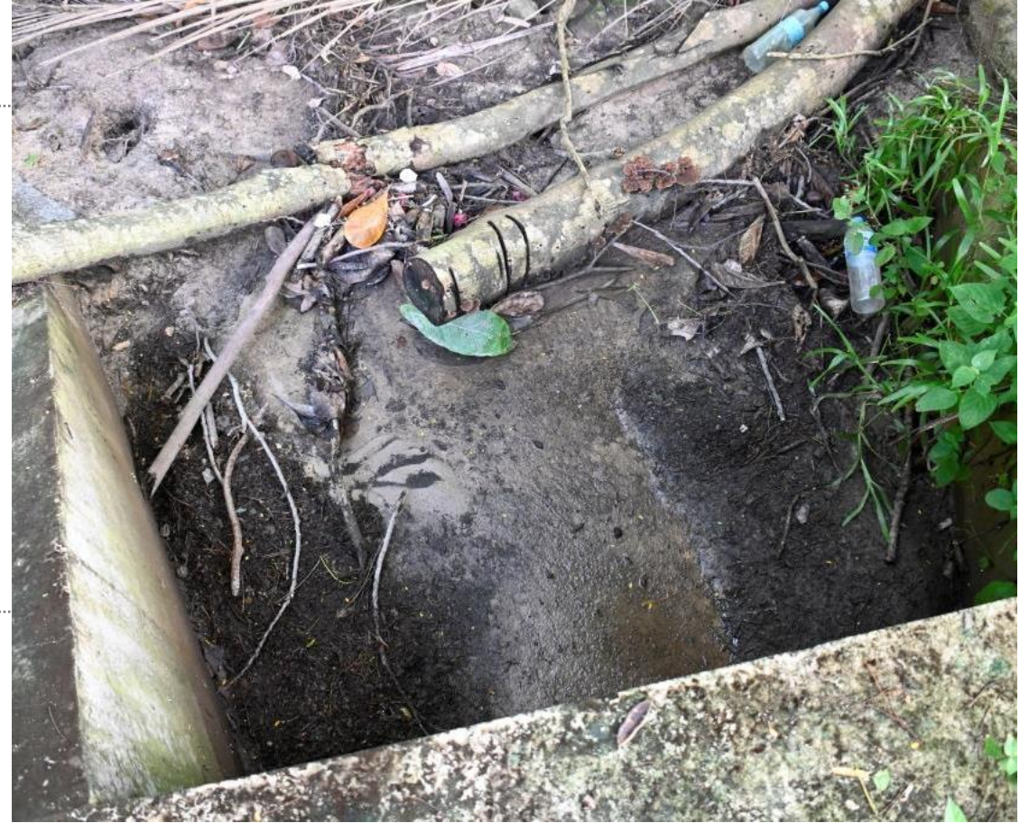
40b. Another sedimentation trap not working
