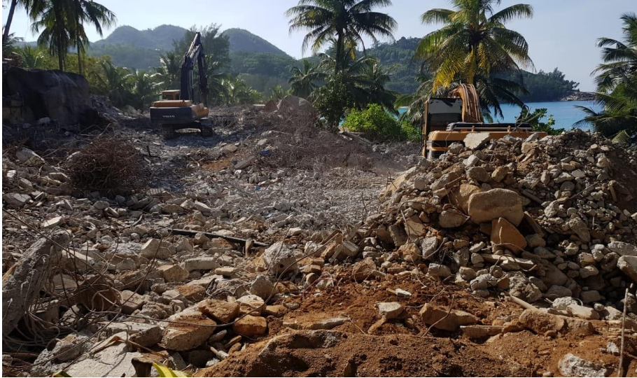
13a. Demolition using heavy machinery
