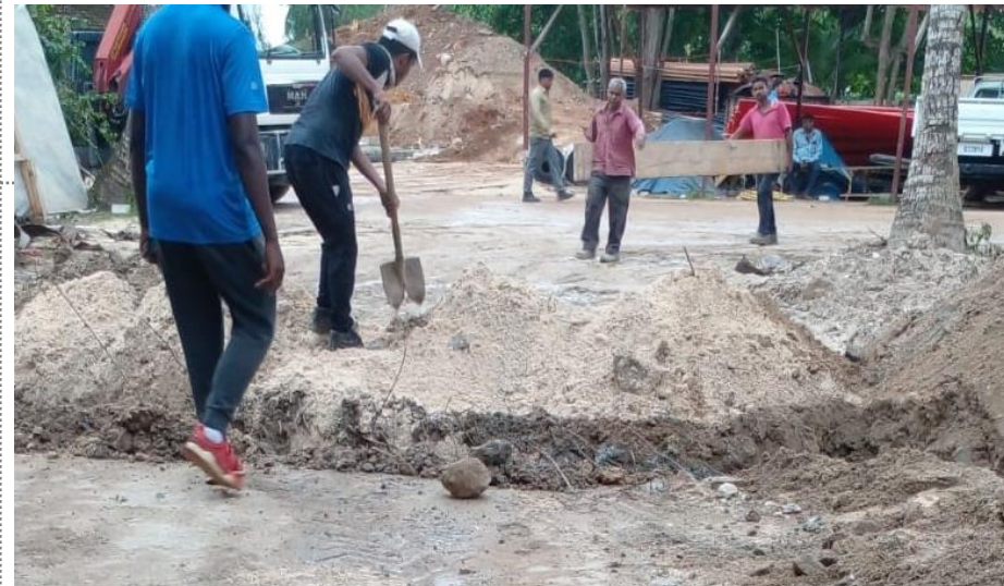
22c. New trench on main road
