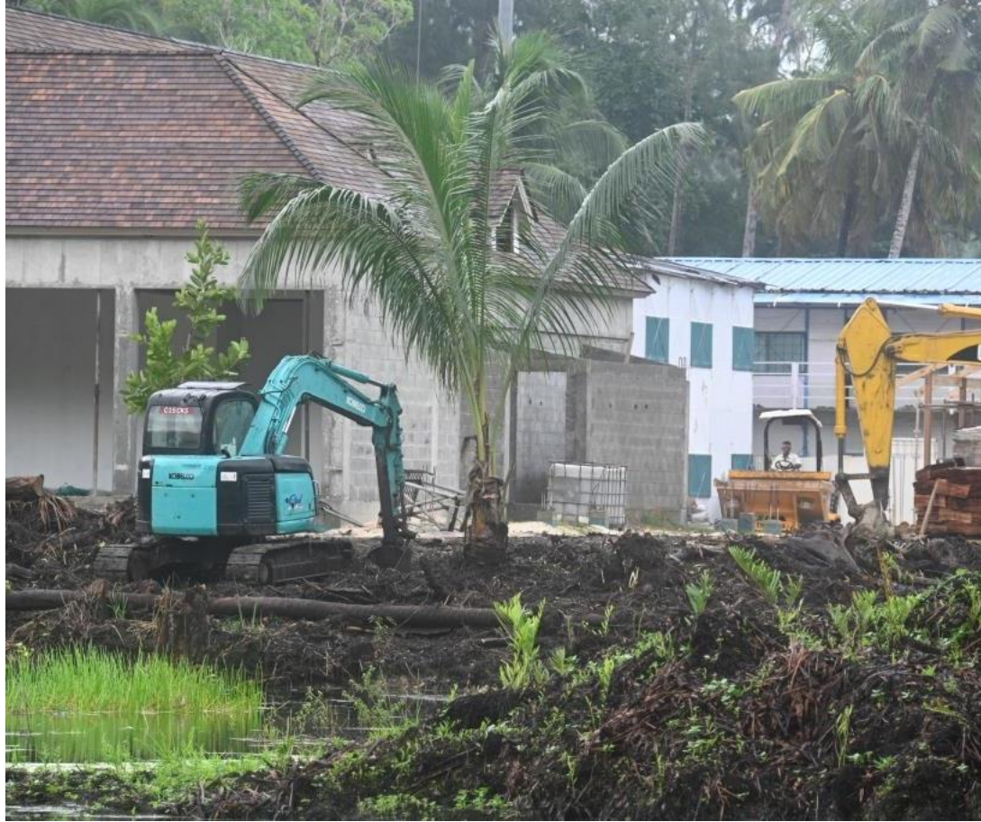
57a Desilting by excavator
