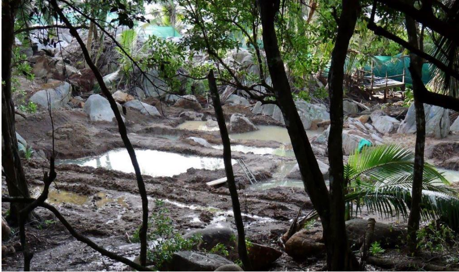
38a New foundation being dug for the new northern hill villas
