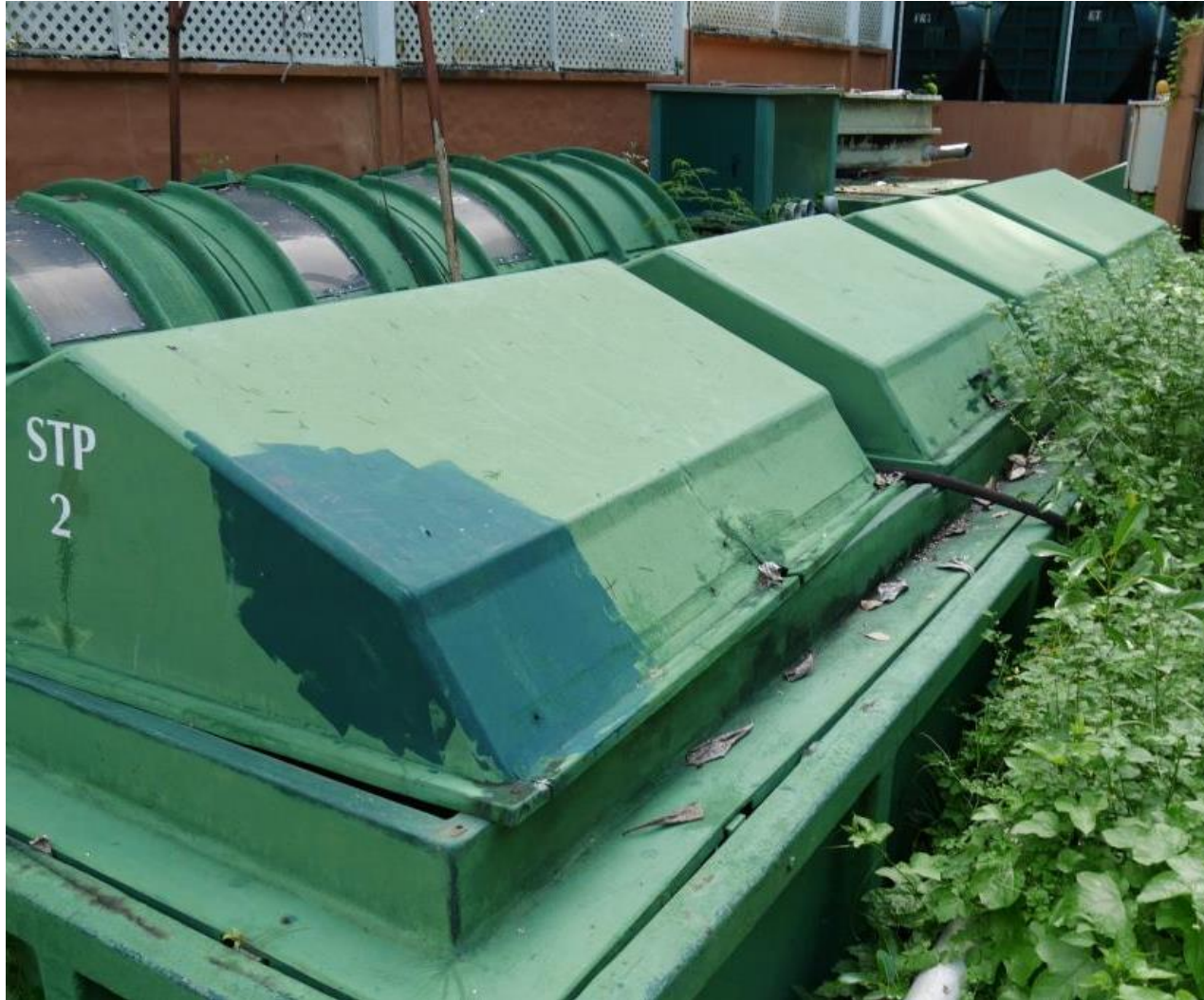
11. One of the old sewage treatment plants demolished in 2020
