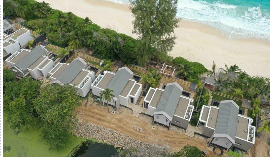
43b All beach villas have the same front garden set up and now the additional eating platforms going out further
