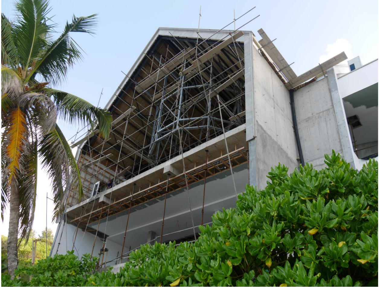
Photo 2: Main lodge seems to have additional height added to the existing structure
