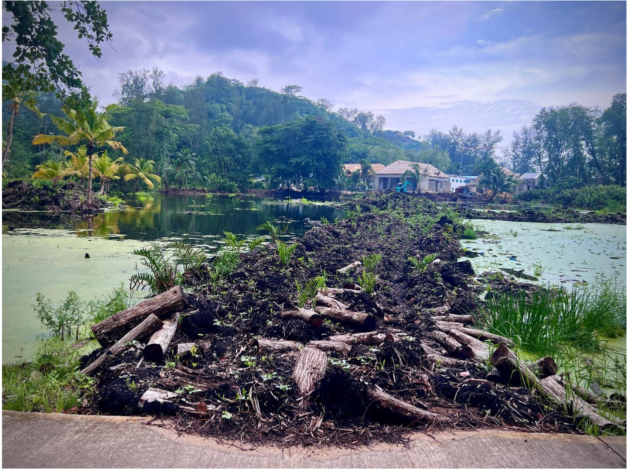
Photo 1: Evidence of dredging activity in the middle of the wetland habitat. Excavator visible in the background (photo taken February 2023)
