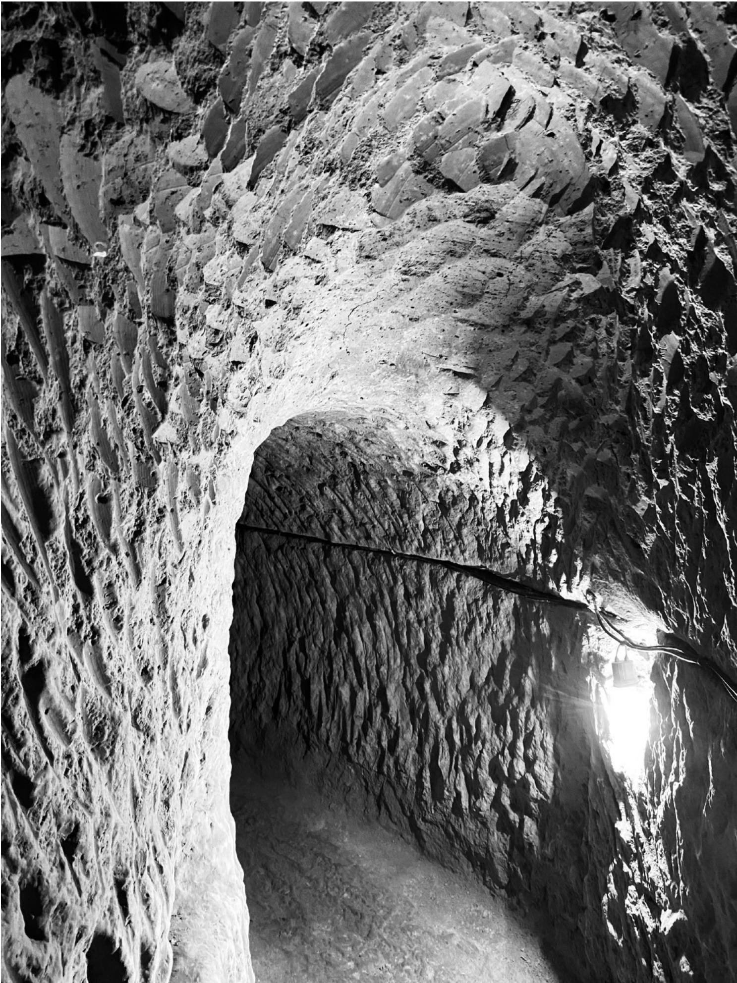
1.2m-tall Tunnel Space Dug with Farming Tools, China, 2023
