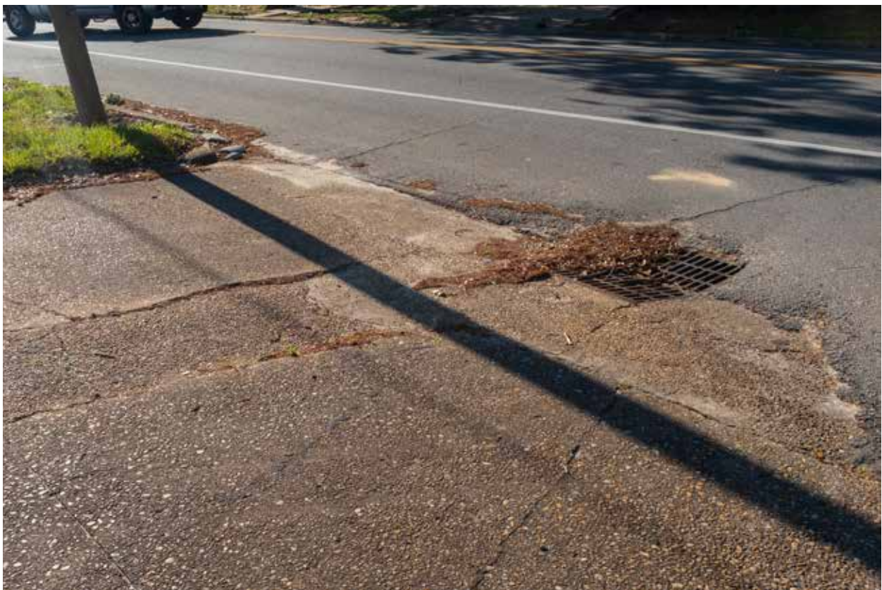
Figure 4.01: Inadequately draining stormwater inlet
