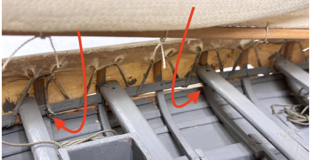
Figure 42. Fill locations between the outermost side stringer and the side ribs on the PL side.
