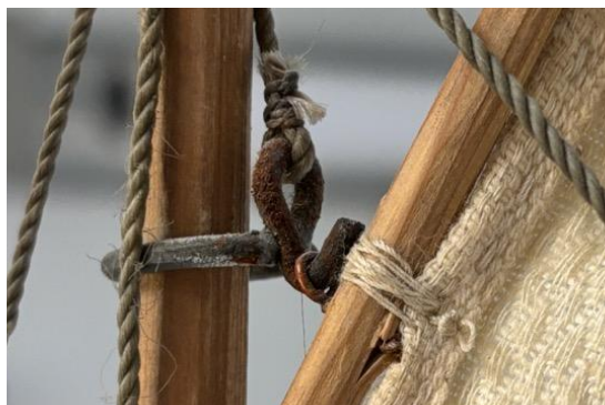
Figure 20. Dark red-brown and white corrosion products, top of the sail.
