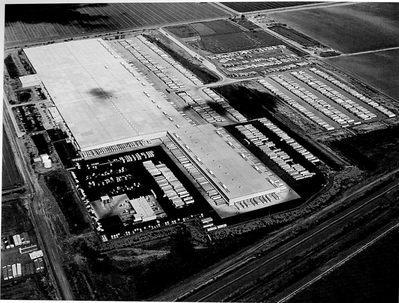
Figure 8. Wal-Mart Distribution Center, Phoenix, Arizona. (Photograph by Alan Berger, 2003–2006)
