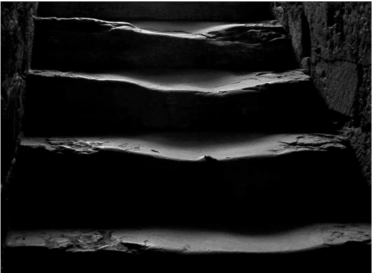
Blackfriars Priory | South Range Staircase.
