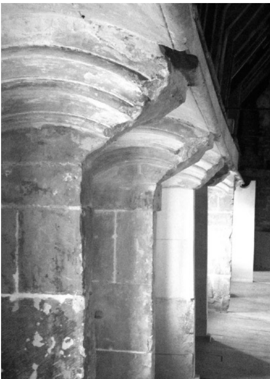
Blackfriars Priory | South Range | Evidence of the buildings industrial past, 13th Century stone cut away to allow for bottling plant machinery.
