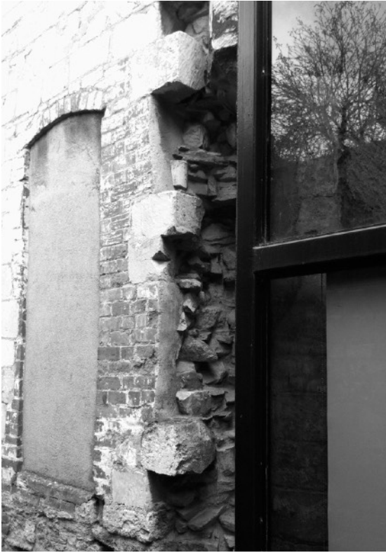
Blackfriars Priory | North Range | Evidence of the 1950's Ministry of Works conservation project.
