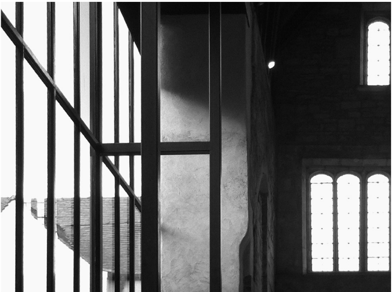
Blackfriars Priory | North Range | Ministry of Works Conservation Project.
